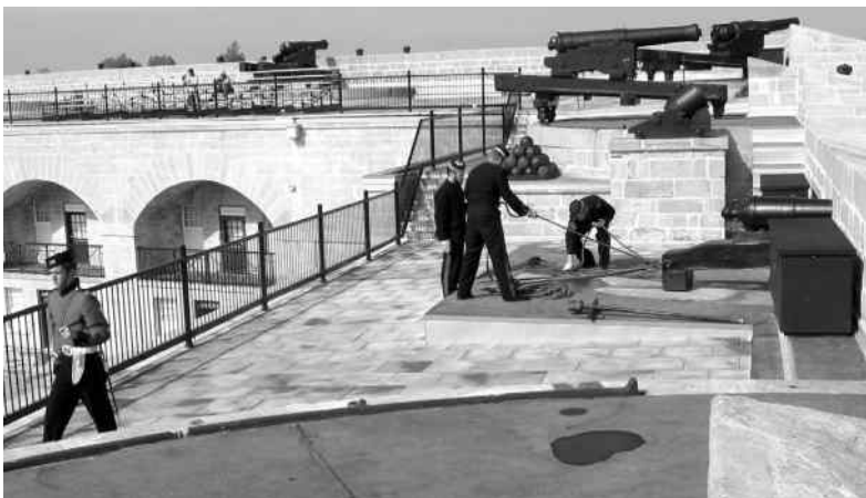
Figure 9. The rehabilitated terreplein above the east officers' casemates, summer 2005. Parks Canada, 2005.
