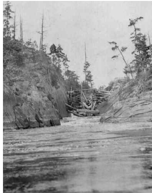
Figure 8. Log water control dam on the Severn River, circa 1860s. The waterlines on rocks show fluctuating seasonal flows. Photo courtesy of Sara Clipsham.
