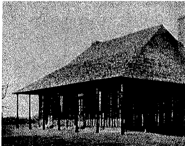
Figure 5: One of the very few French post-on-sill buildings on this continent, at Cahokia, Illinois, built ca. 1737. The posts are of dressed timber and spaced apart, however, at Sainte-Marie I, they would have been undressed and spaced closer together. Note the two chimneys offset to the roof ridge. The roof, with its flared projecting eaves extending into a verandah was an eighteenth-century development.
