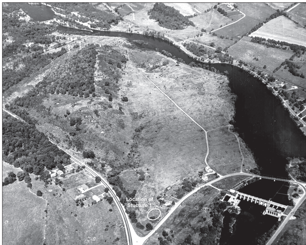
Figure 13. Nassau Mills in 1964, looking north. Source: Trent University Archives.
